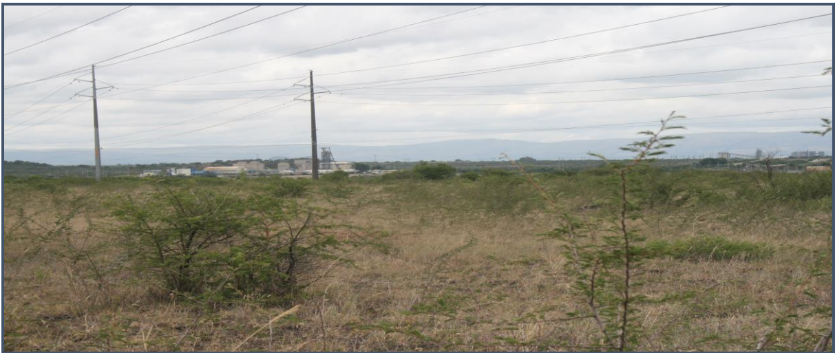
Figure 27: Mine infrastructure can be seen from the substation site
